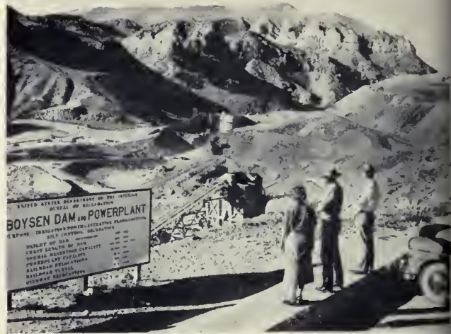
BUILDING BOYSEN —An important key to the development of the Wind River Basin. Photo by T. R. Broderick, Region 6.
